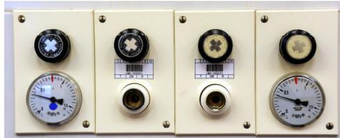
*Fig. 16-1 Central oxygen distribution panel
